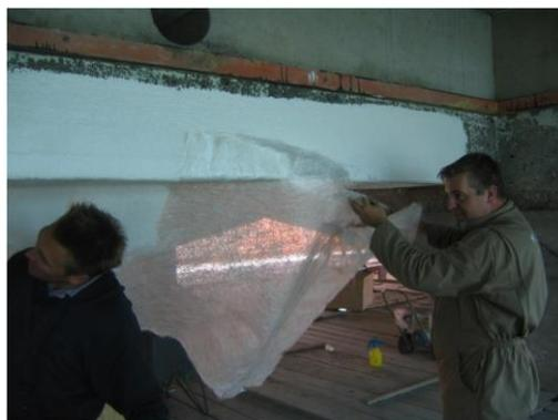
2. Or a fibreglass tape with coarse (8 x 8) mesh of appr. 10cm width in the first layer of fresh coating/waterproofing, to act as a reinforcement along the joints.
