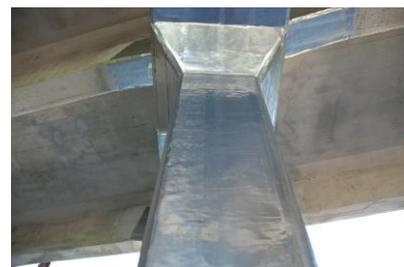
In case no waterproofing system will be applied it is recommended to seal all the exposed ends to avoid humidity ingress.
