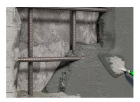
Before applying the mortar saturate the concrete surface with clean water. Substrate should be saturated but surface dry with no standing water.
