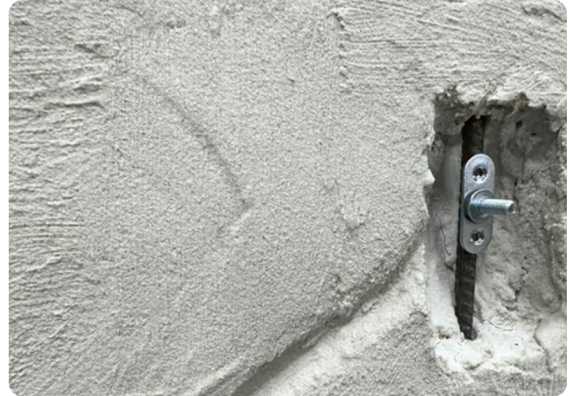
Step 8. Use durable connections to the reinforcement.
