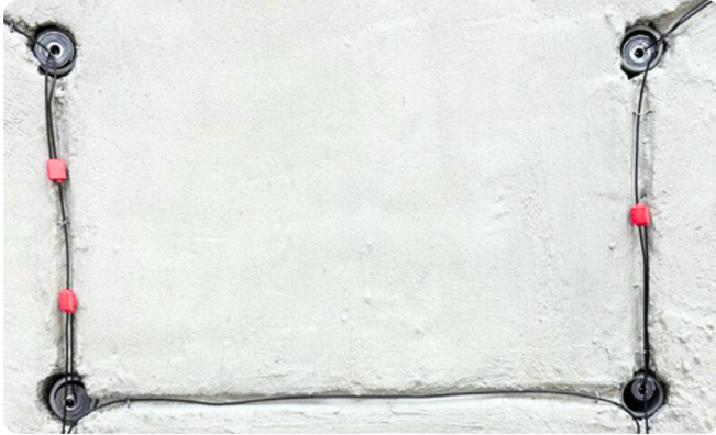
Step 7. Interconnect anodes via anode wire and secure with wire crimps.
