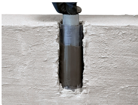
Step 4. Insert anode into borehole, leaving ~1 cm gap at the end.
