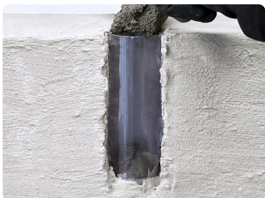
Step 3. Fill with mortar to secure the anode and ensure electrolytic contact.
