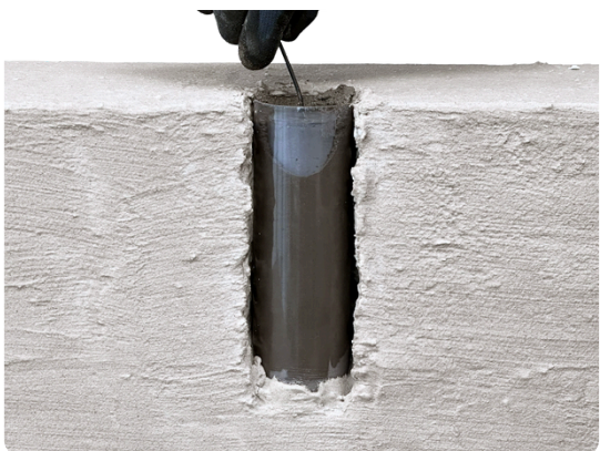
Step 5. Allow mortar to cure around the Galvex DI before closing the hole.
