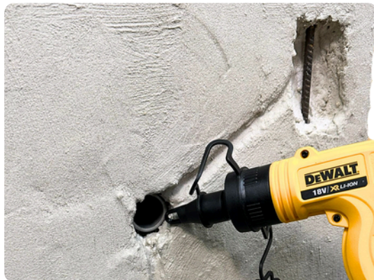
Step 2. Clean boreholes: blow out dust, rinse and keep slightly moist (not dry).
